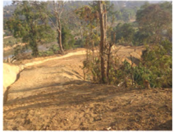
Road Formation from Longtharai Charra to Bhgyamani RP (NREGA)
