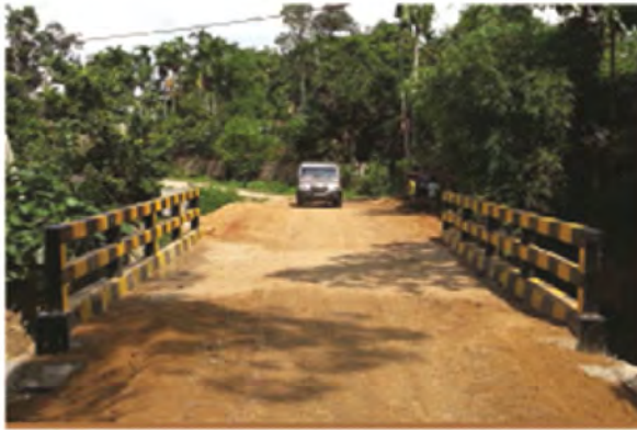
Construction of Box Culvert over Longtarai Chara at Saha Colony (NREGA)
